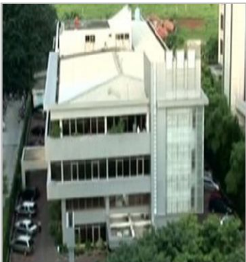
(RASUNA) GRAHA BINAKARSA
