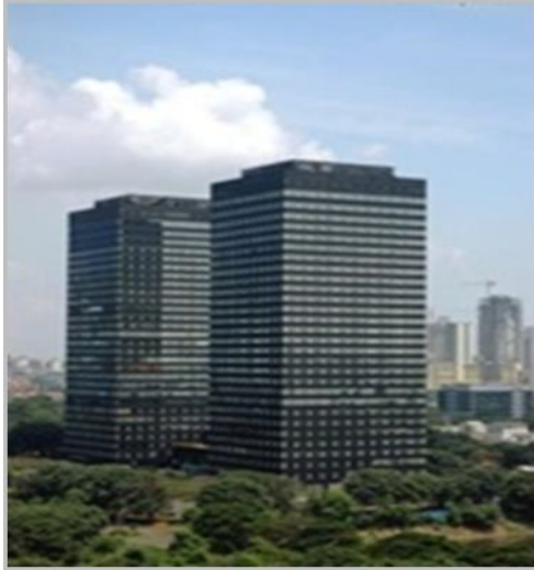
( SUDIRMAN ) LANDMARK TOWER
